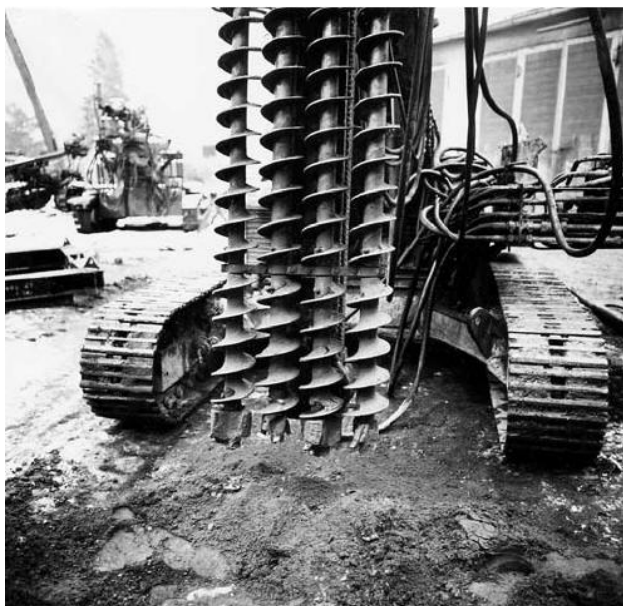
Fig. 7. The first application of Mixed-in-place (MIP) piles, (Stocker and Seidel, 2005).
