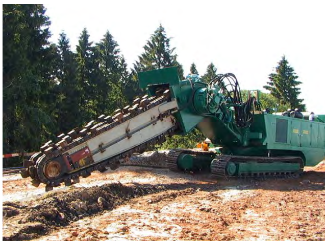
Fig. 13. Trenching machine for construction of walls by deep mixing.
