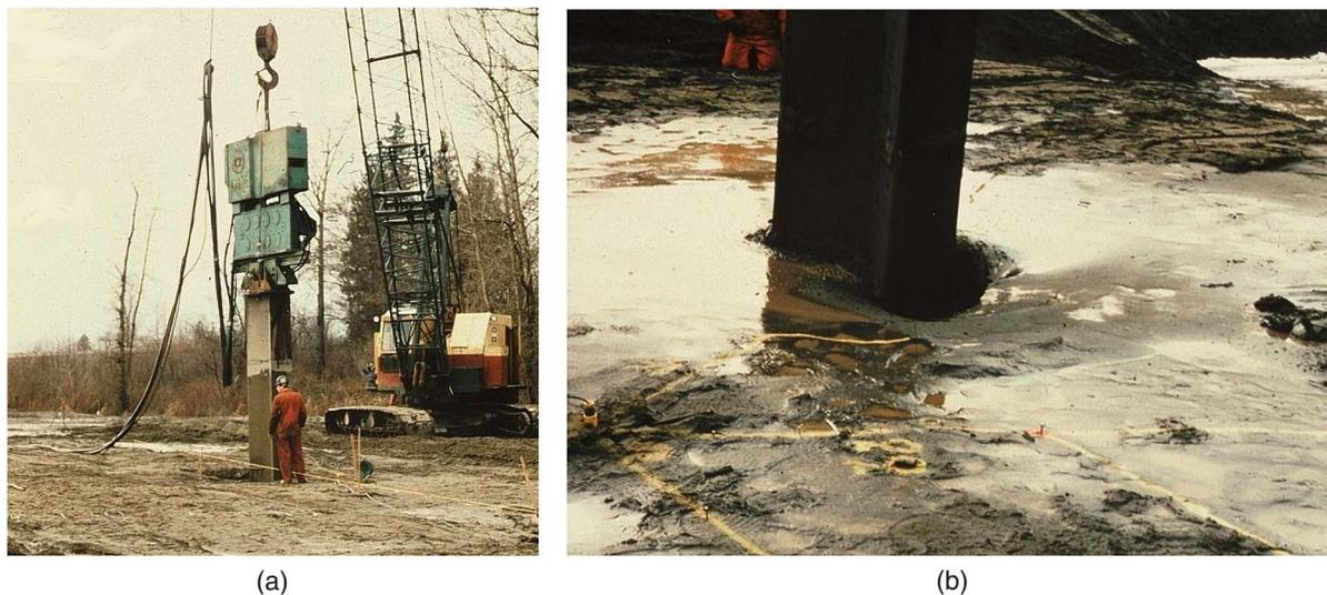
**Fig. 5.** Resonance compaction and liquefaction of zone around Tri Star probe: (a) compaction equipment; and (b) manifestation of liquefaction during resonance compaction. (Reprinted from Massarsch and Vanneste 1988.)
