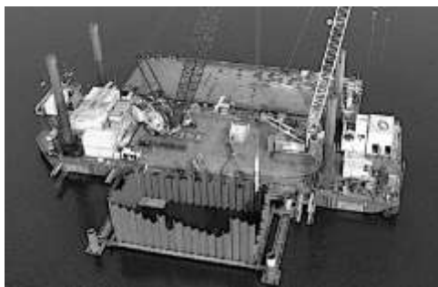
Figure 1. Steel caisson in foreground and barge with pile driving and compaction equipment in background.
