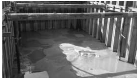
Figure 11. Compacted surface after dewatering of steel caisson. The probe insertion points can be detected.
