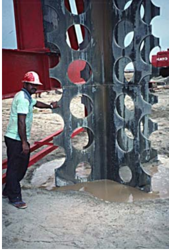
Fig. 13. Liquefaction of water-saturated sand during the initial phase of compaction. Note that the ground water level is 4.5 m below the ground surface.
