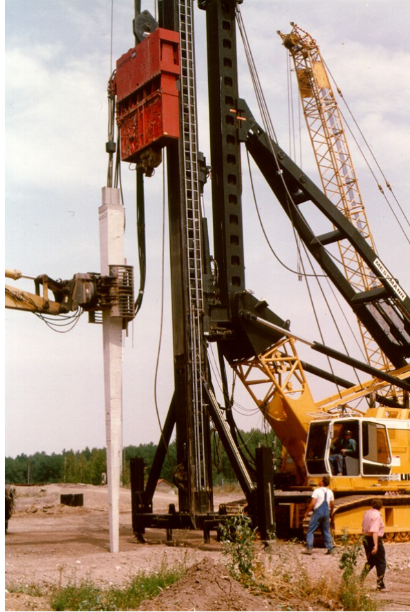
Fig. 11. Installation of conical concrete elements by vibrator with variable frequency.
