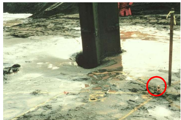
Figure 5. Liquefaction of a zone surrounding the TriStar probe during resonance compaction. The geophone (in circle) installed at 1 m away from the compaction probe
