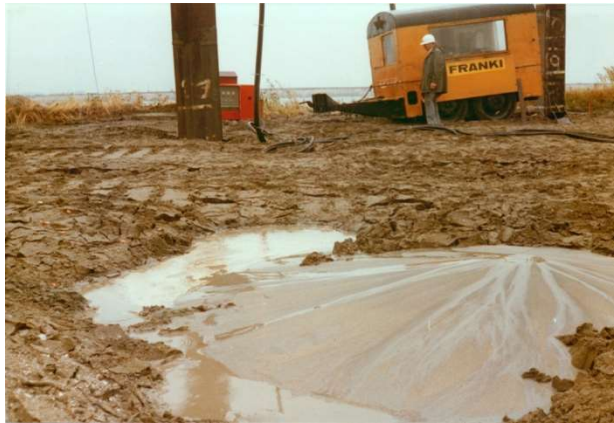
Figure 1. Liquefaction caused by TriStar soil compaction at Borechem (Wallays 1982).
