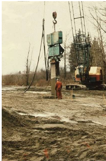
Figure 3. Resonance compaction at Annacis Channel, Vancouver by TriStar probe with variable frequency vibrator
